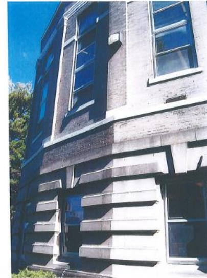
Rear of building showing upper windows. It is the upper portion of the rear exterior that is in critical need of rehabilitation due to rusting steel lintels
